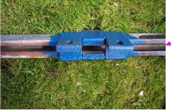
the top part of the tower this is where the guy rope from the ground anchors will be tied to.
