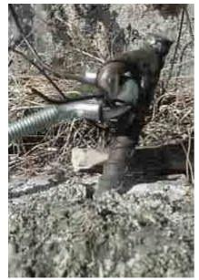
These types of ground anchors are easy to make as they are simple glued into the ground. At Mr Bigins location there is soft soil so a ground anchor called a 'dead man' will have to be used basically there is a weight under the ground which is pulled on to when the tower starts to move in strong winds etc.
