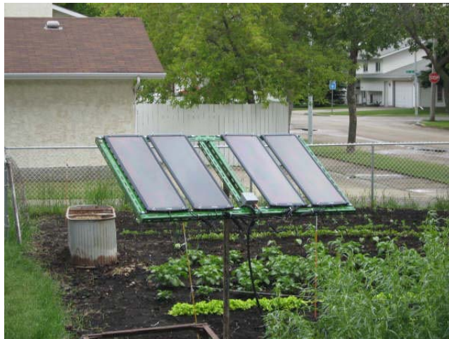
Illustration 6: Overall front view of completed frame.
